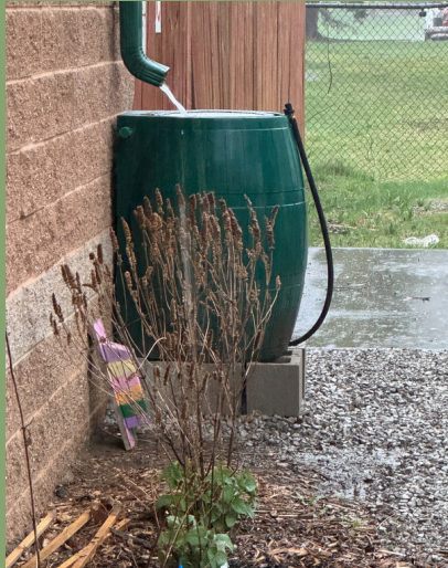
Rain Barrel Project @ Stage
