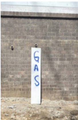
Meter location marked with plywood marked Gas.
