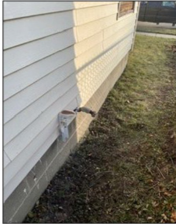
New meter location visible with stubbed out fuel line.
