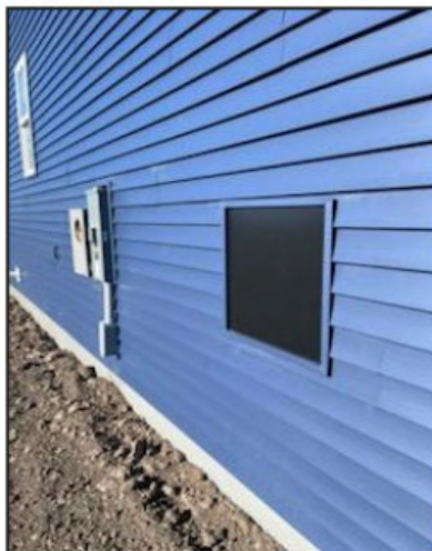
Weatherproof permanent backer plate for mounting a meter.
