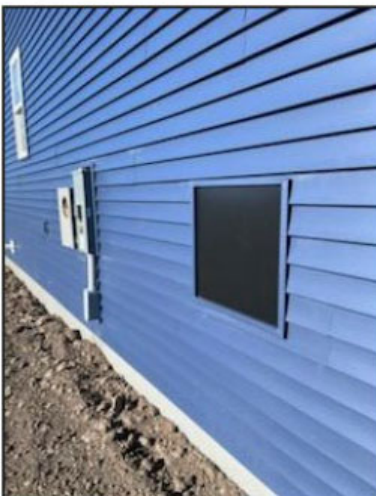
Weatherproof permanent backer plate for mounting a meter.
