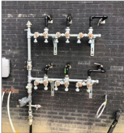
Multi-meter bracket showing Consumers Energy tags on fuel lines and service line connected to bracket.
