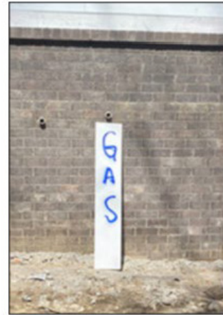
Meter location marked with plywood marked Gas.
