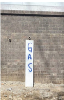
Meter location marked with plywood marked Gas.
