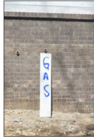
Meter location marked with plywood marked Gas.
